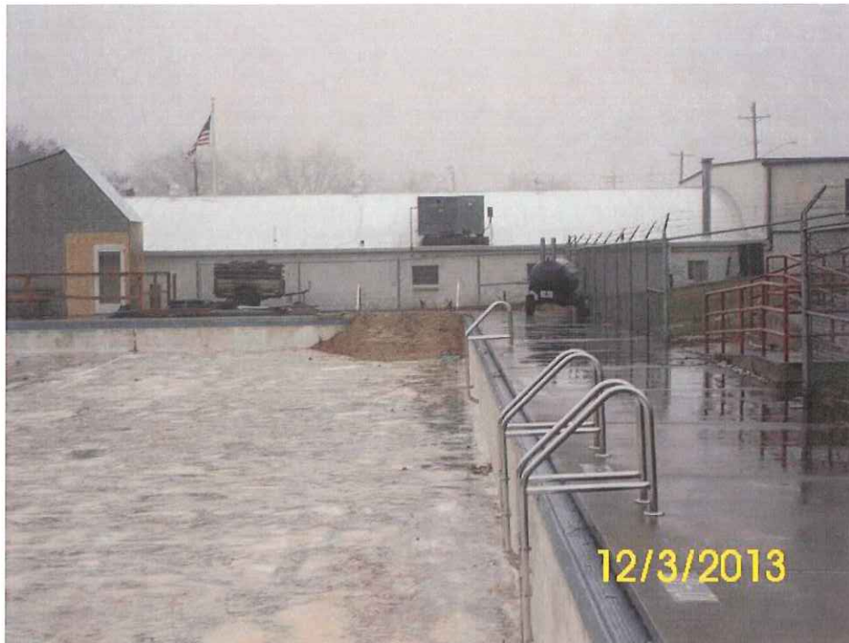
Shallow Area - Staircase filled in with Aggregate
