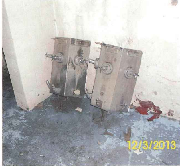
Existing Dismantled Showers
