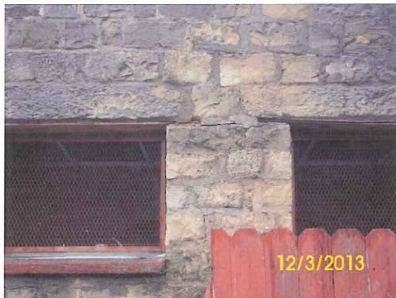
Lintels – Replacement required, bowed, rusted, unsafe
