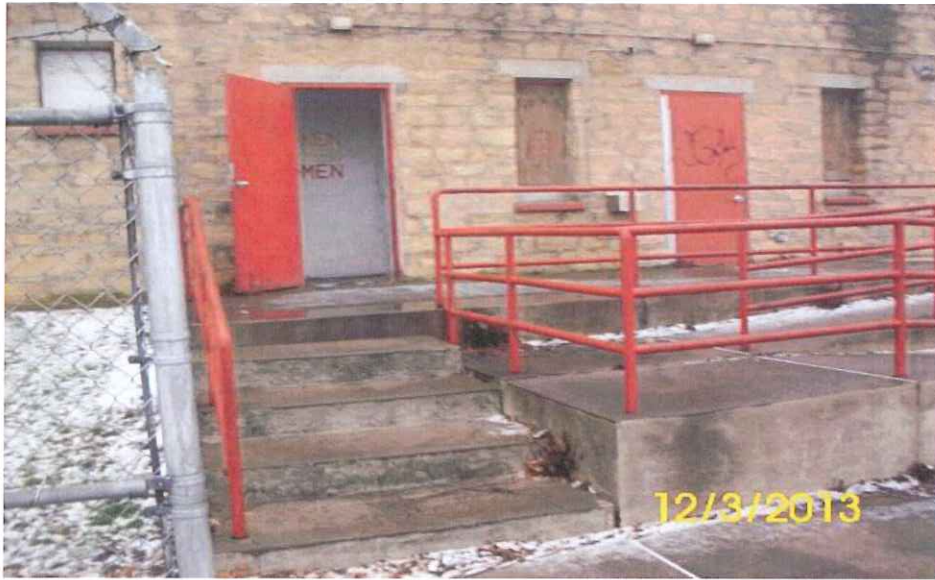
Stairs to bathhouse
