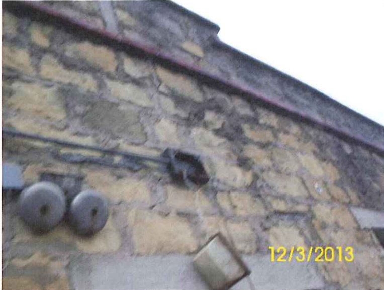
Bathroom exterior lighting
