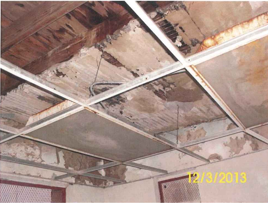
Ceiling and Roof Deck
