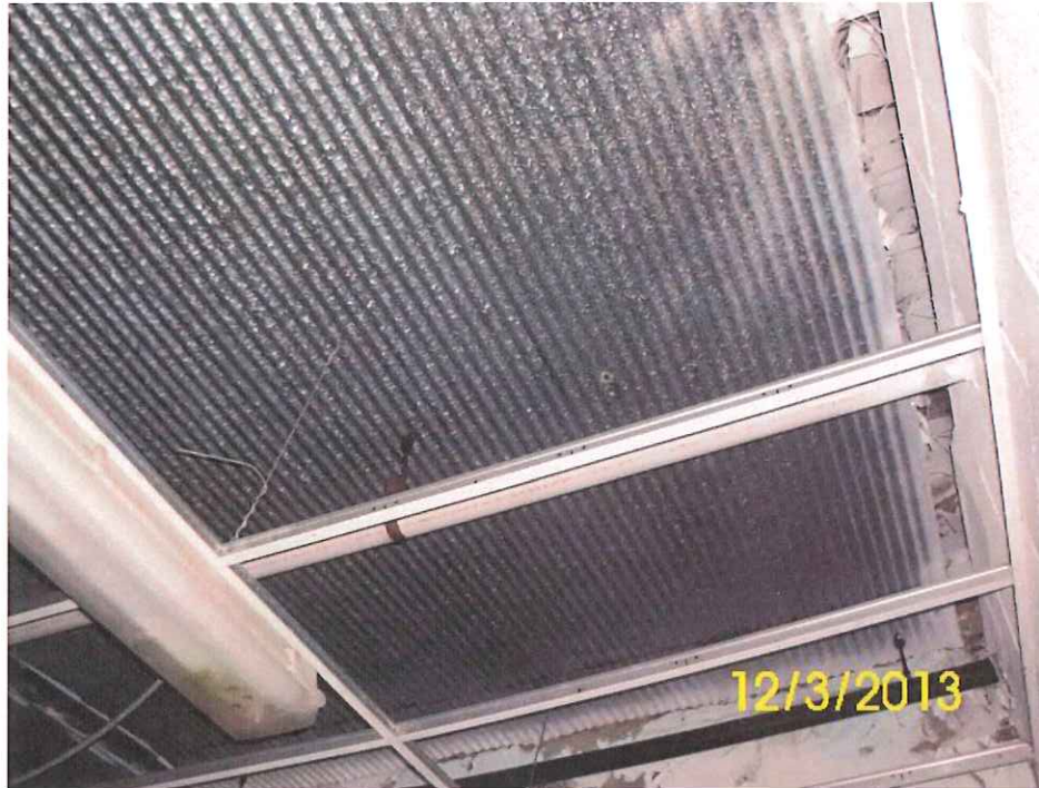
Ceiling with steel underside attached to Wood Rafters
