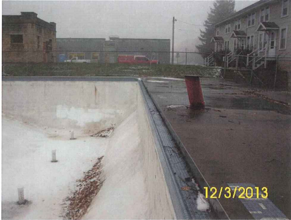
Main Drains and Diving Tower Column
