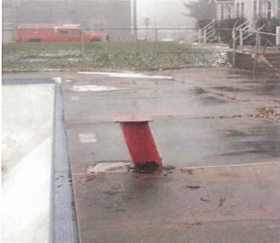
Diving Tower Removed Pedestal Remains
