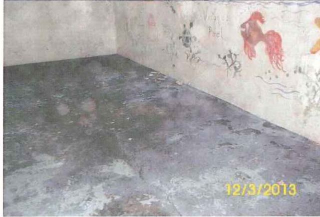
Bathroom – Floor and wall
